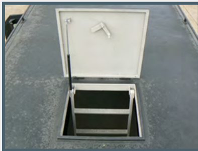
Roof Hatch Integrated roof hatch in the rear cabin with ladder, provides easy roof access
