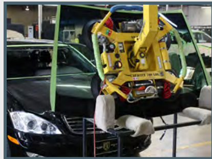
Using robotic equipment to install the armored glass.
